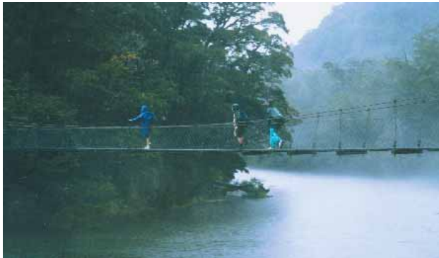
Swing bridge over the Arthur River
